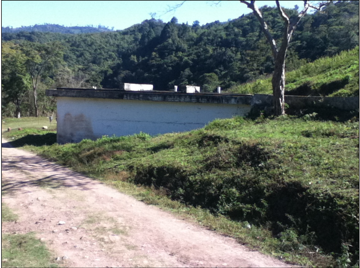
Figure 2.14: Location of Imhoff Tank in Reference to the Road (Walker 2011)
