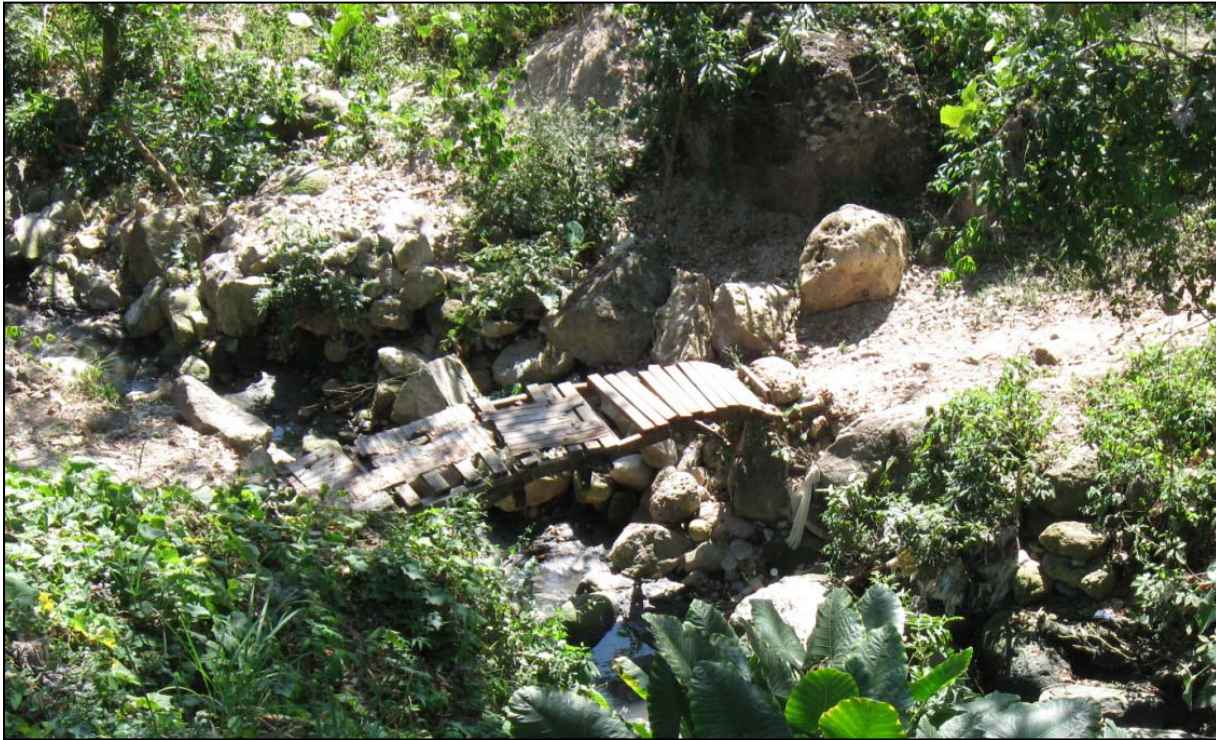
Figure 2.37: Human Traffic Bridge Located Below the Imhoff Tank (Walker 2011)
