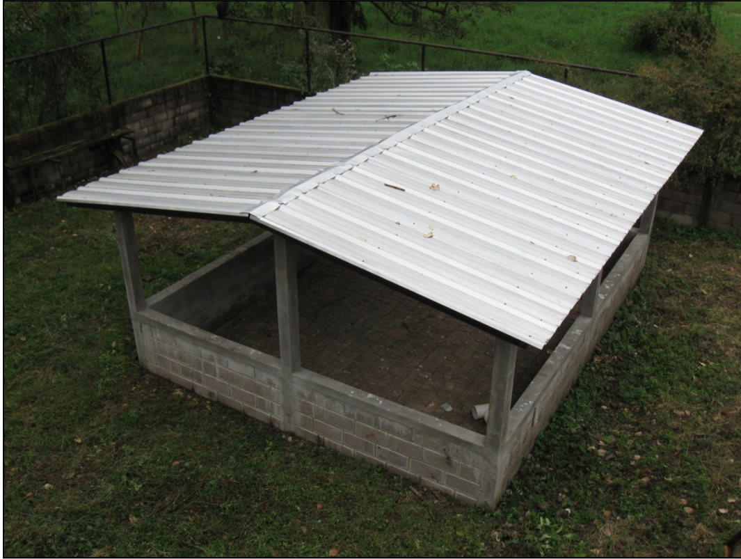
Figure 3.17: Las Casetas Sludge Drying Bed as Constructed (Puckett, 2011)
