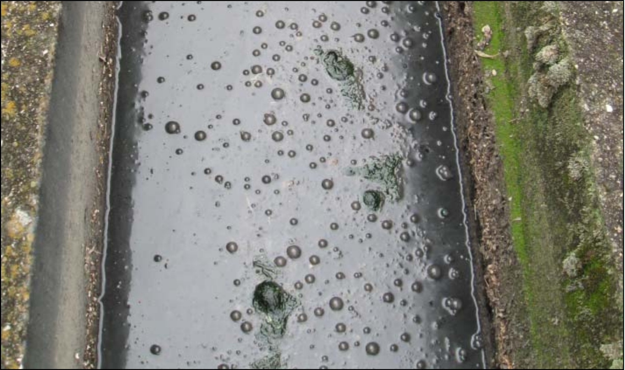
Figure 2.23: Scum Channel after Cleaning (Walker 2011)
