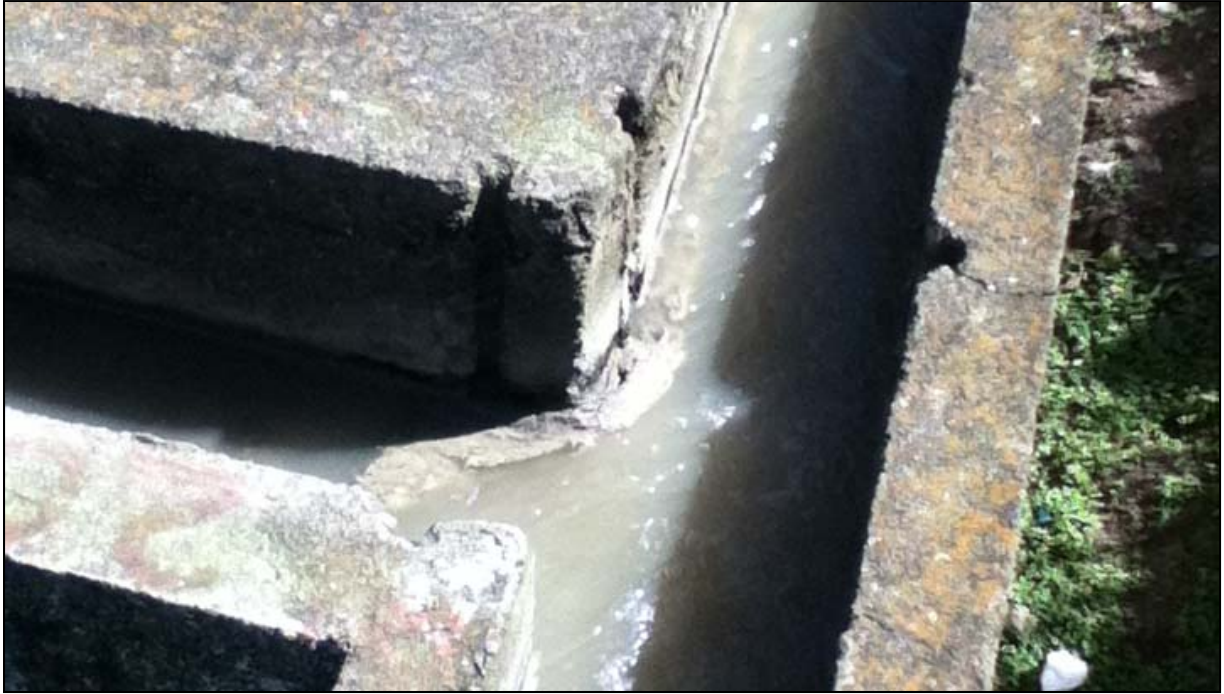
Figure 2.15: Control Flow Gate Slots (Walker 2011)
