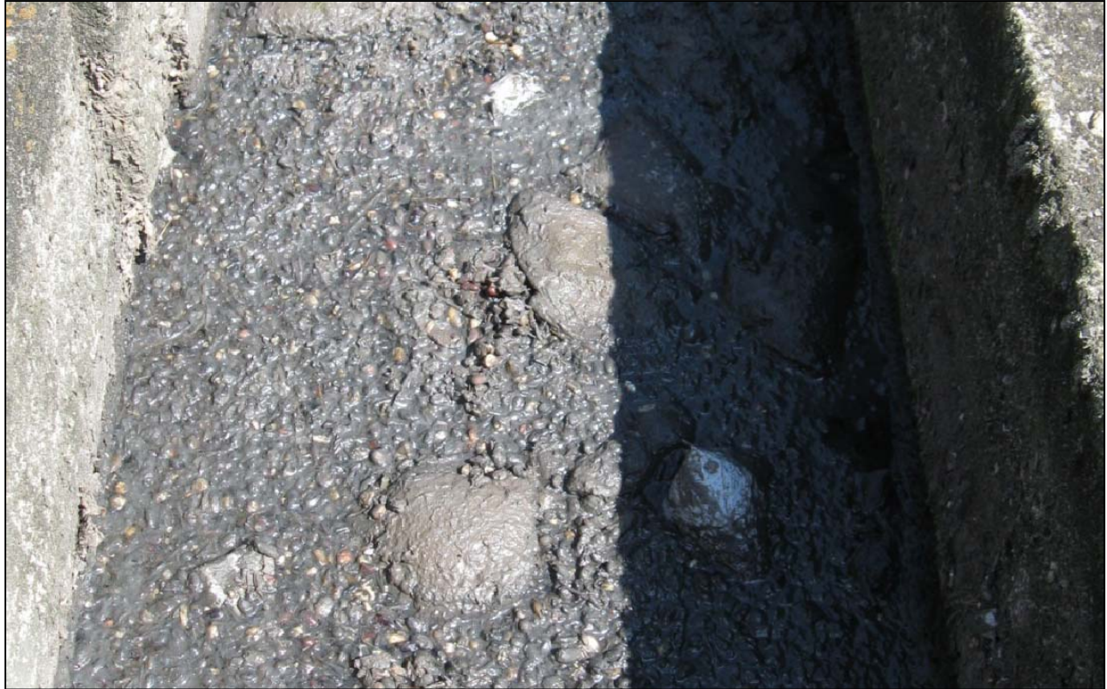
Figure 2.22: Scum Build-up in Channel (Walker 2011)
