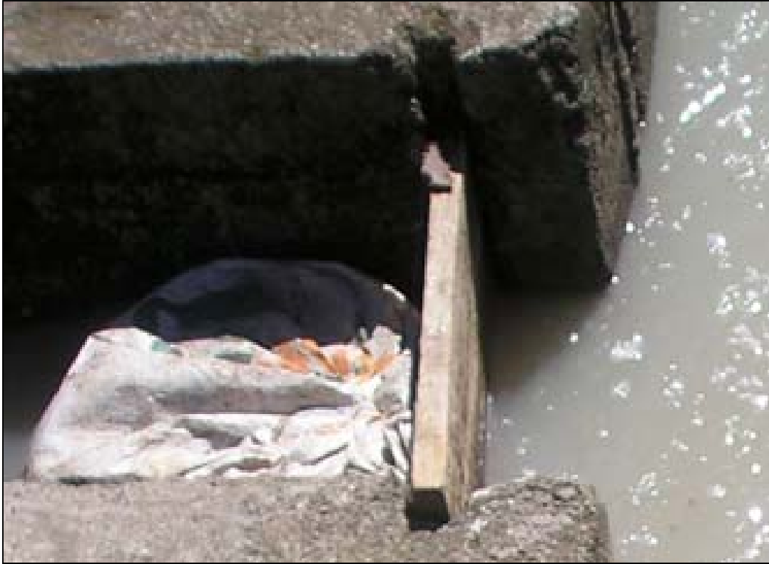
Figure 2.17: Control Flow Gate with Sand Bag to Create a Tighter Seal (Mikelonis & Hodge, 2008)
