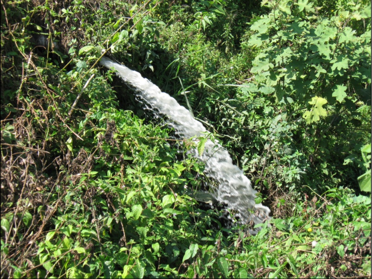
Figure 2.24: Effluent Pipe from the Las Vegas Collector System (Walker 2011)
